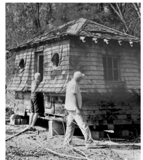
Jack Conlon and Greg Titus working on the trolley barn restoration.
